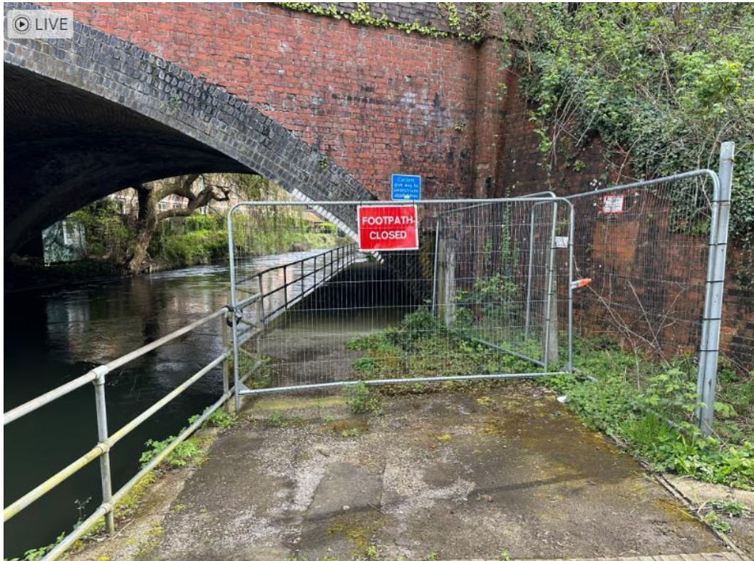
Image: blocked access along the Avon Valley Path
